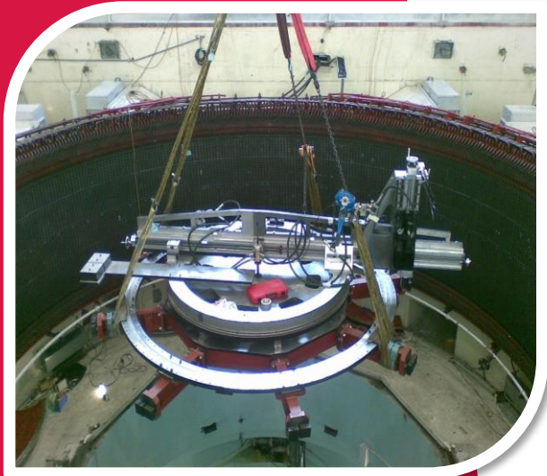
The adapted Mirage MM1875ie being moved into position.
