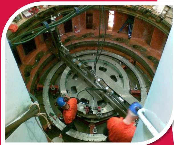
The machine is rested onto a support platform and clamped into position using the 8 legs and adjustable jaws.
