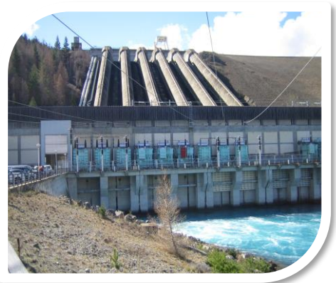
The Benmore Dam in New Zealand
