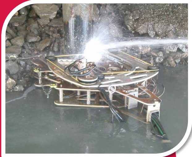
The DWS in action on the project.
