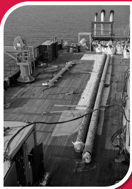
The first two pipe sections recovered from the sea bed.
