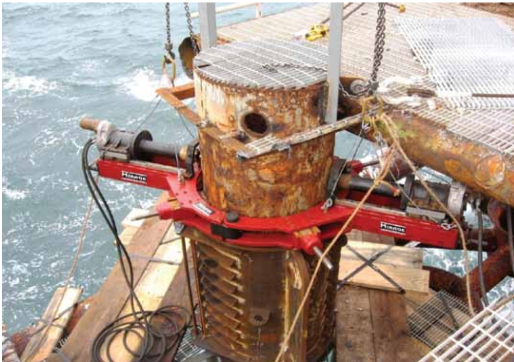
The DDU1636 machine installed – drilling 6" pins.
