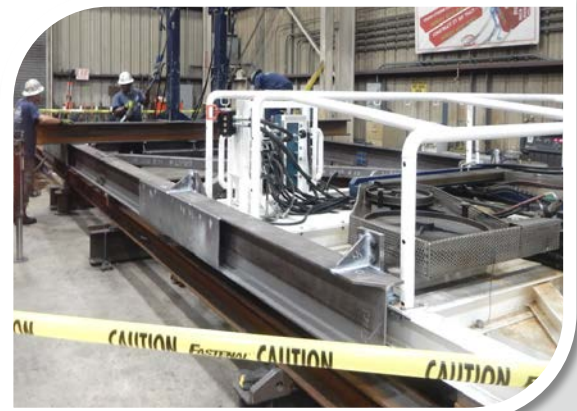
Above: The whole assembly mounted into the cantilever frame.
